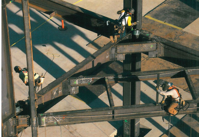
▲ Steel erection for the School of Engineering Library.
