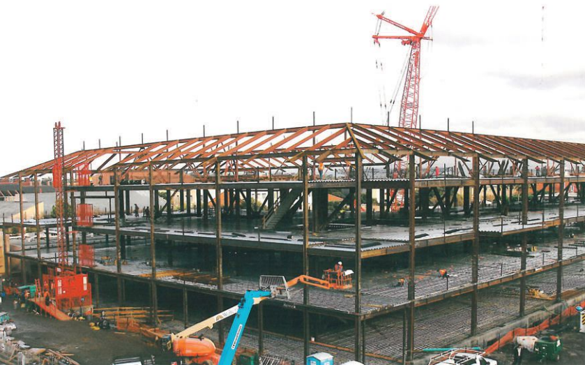
◀ Framing for the Environment and Energy Building, which used 1,470 tons of steel in all.
